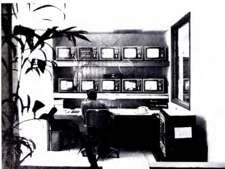
Dispatcher-customer relations desk takes all service calls, sends out service crews, watches all cable channels for proper operation.
