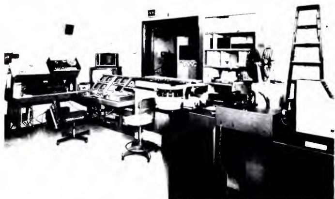
Cable control room, next to two-story studio, has switching in front of studio window. Norelco LDH-1 film chain at the right. IVC 1-inch and Sony 3/4-inch cart machines are primary sources of recorded video programming.
